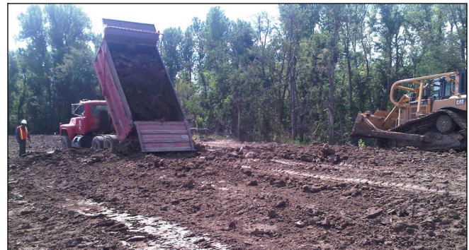
Crews resumed work at the lower crevasse yesterday evening after heavy rain and lightning Wednesday caused a temporary work stoppage.
