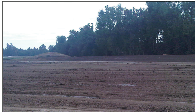
A nearly-complete levee segment at the upper crevasse. This weekend, quality assurance inspectors will verify that this segment complies with our requirements for interim elevation and cross section.
