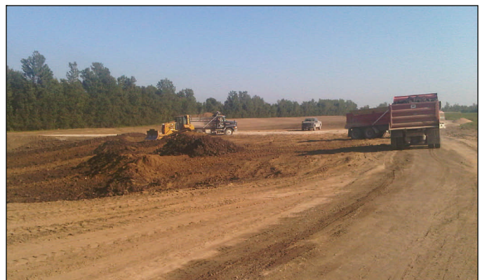
Placing clay into the third of five scour holes Monday. Crews previously filled the holes to the water table with sand, and are now placing clay in the hole to provide a stable base for the levee and to resist seepage.
